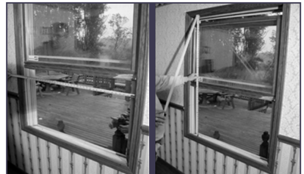
The jamb depth for a Garden window should be measured from the very most interior wall surface to the very most exterior wall surface.
